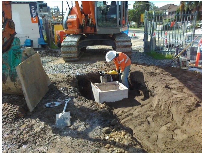
Compaction of backfill around pit
