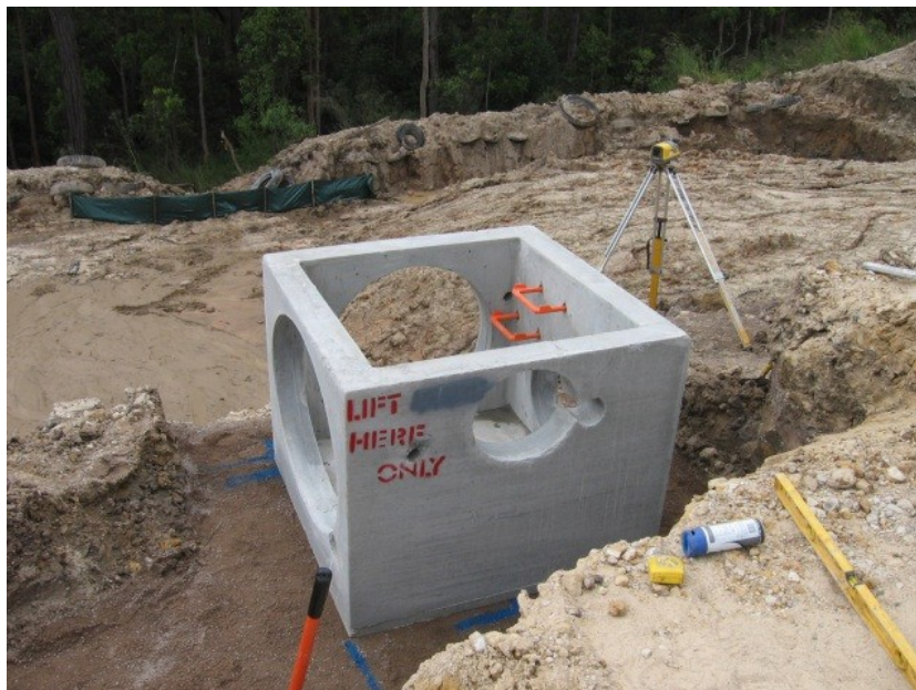
Pit positioned on leveled bedding material
