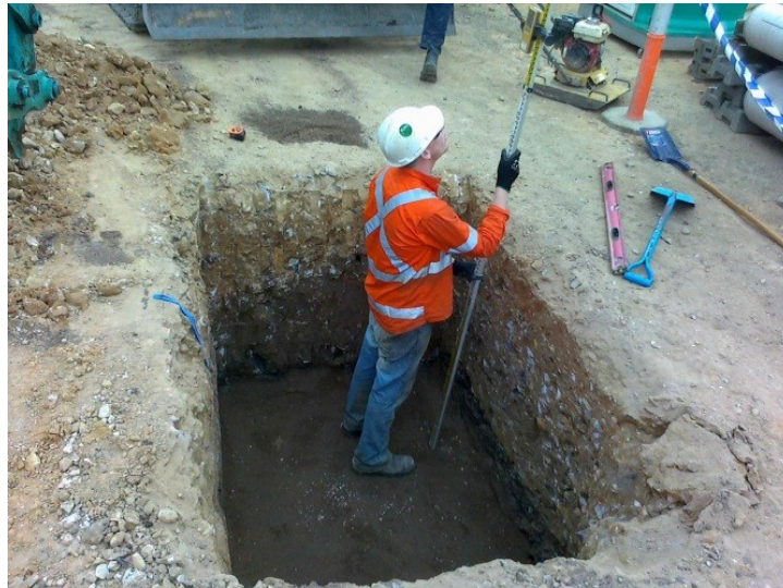
Checking the base
