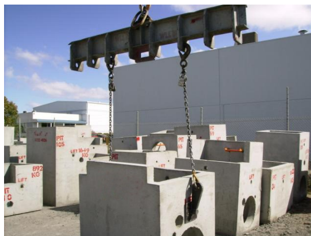
Lifting with spreader bar
