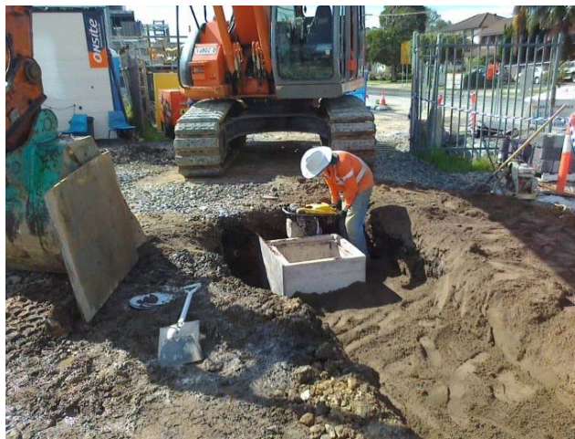
Compaction of backfill around pit
