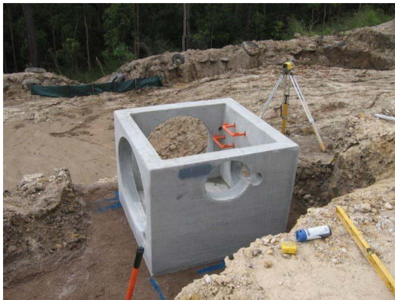
Pit positioned on leveled bedding material
