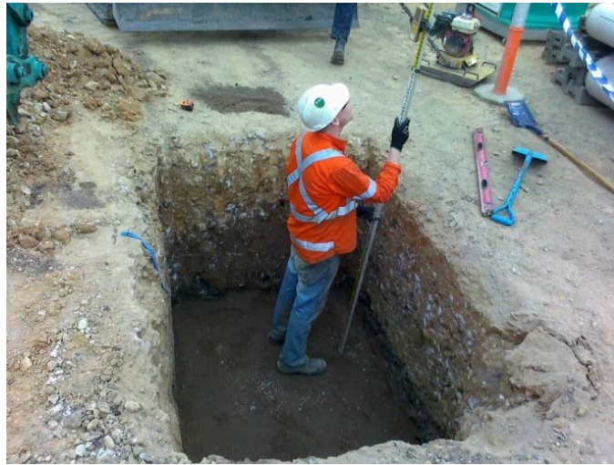
Checking the base
