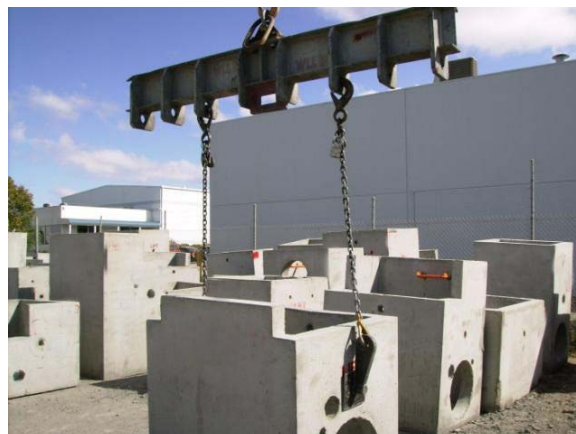
Lifting with spreader bar
